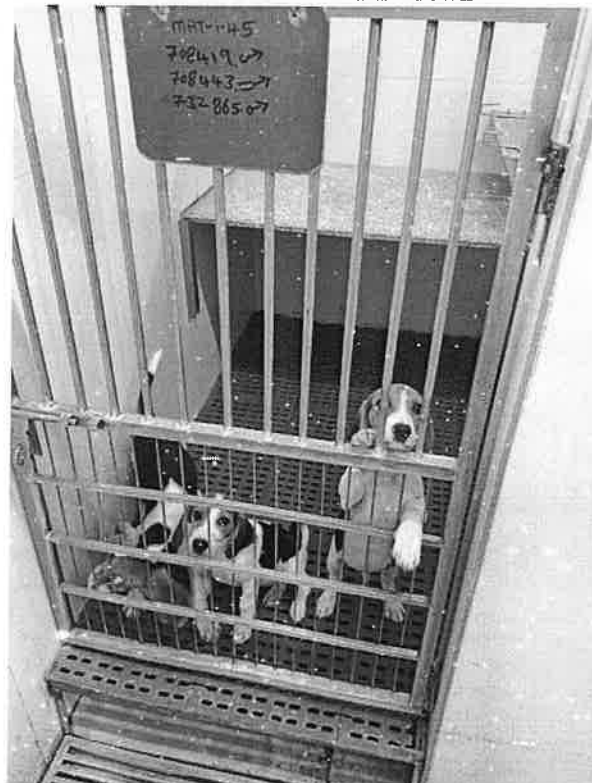
Photo 12: Polymer flooring with drainage channels, making it uncomfortable for animals to stand or lie down
