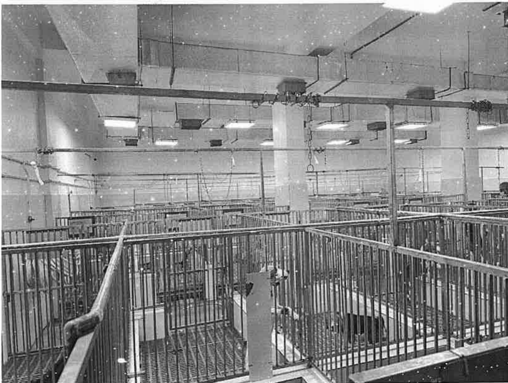
Photo 24: Enclosed space lacking natural light and enrichment
