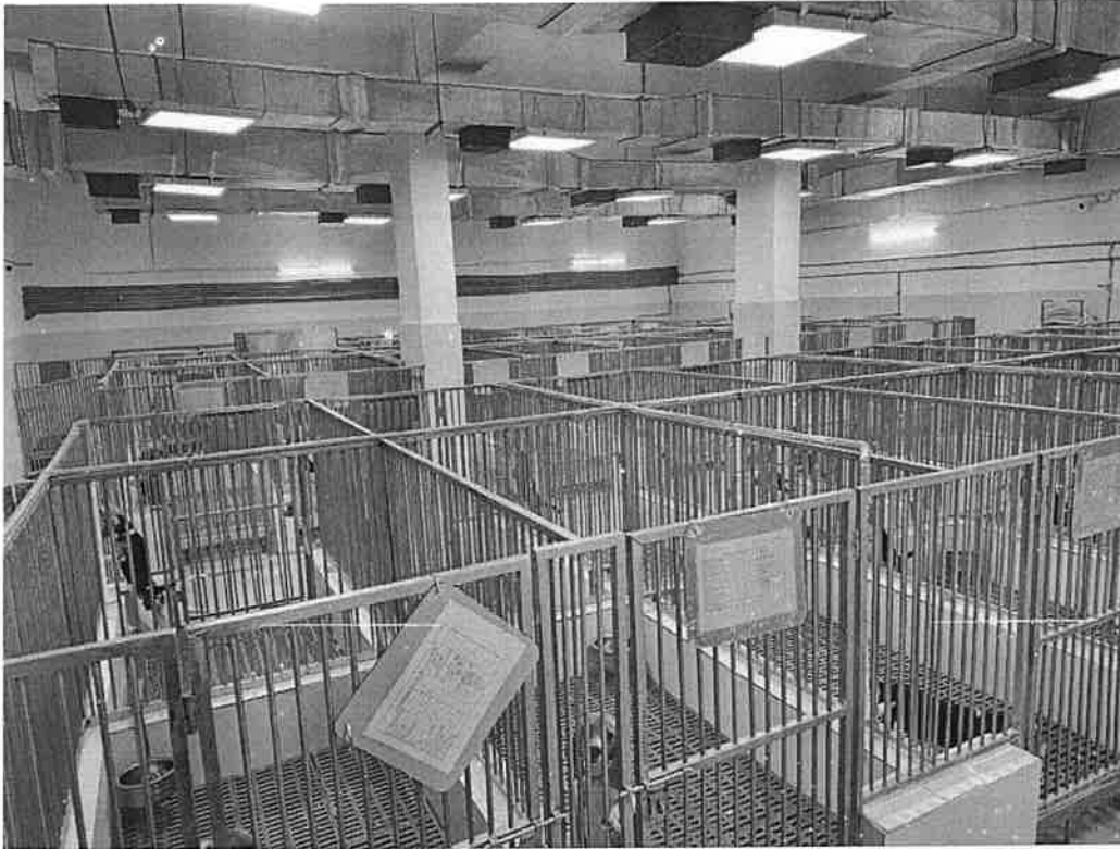
Photo 23: Enclosed space lacking natural light and enrichment
