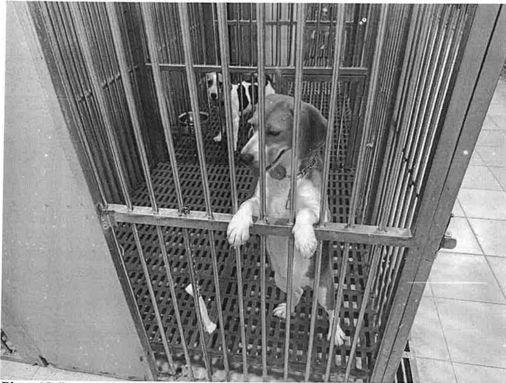
Photo 15: Polymer flooring with drains, uncomfortable for animals to stand or lie down
