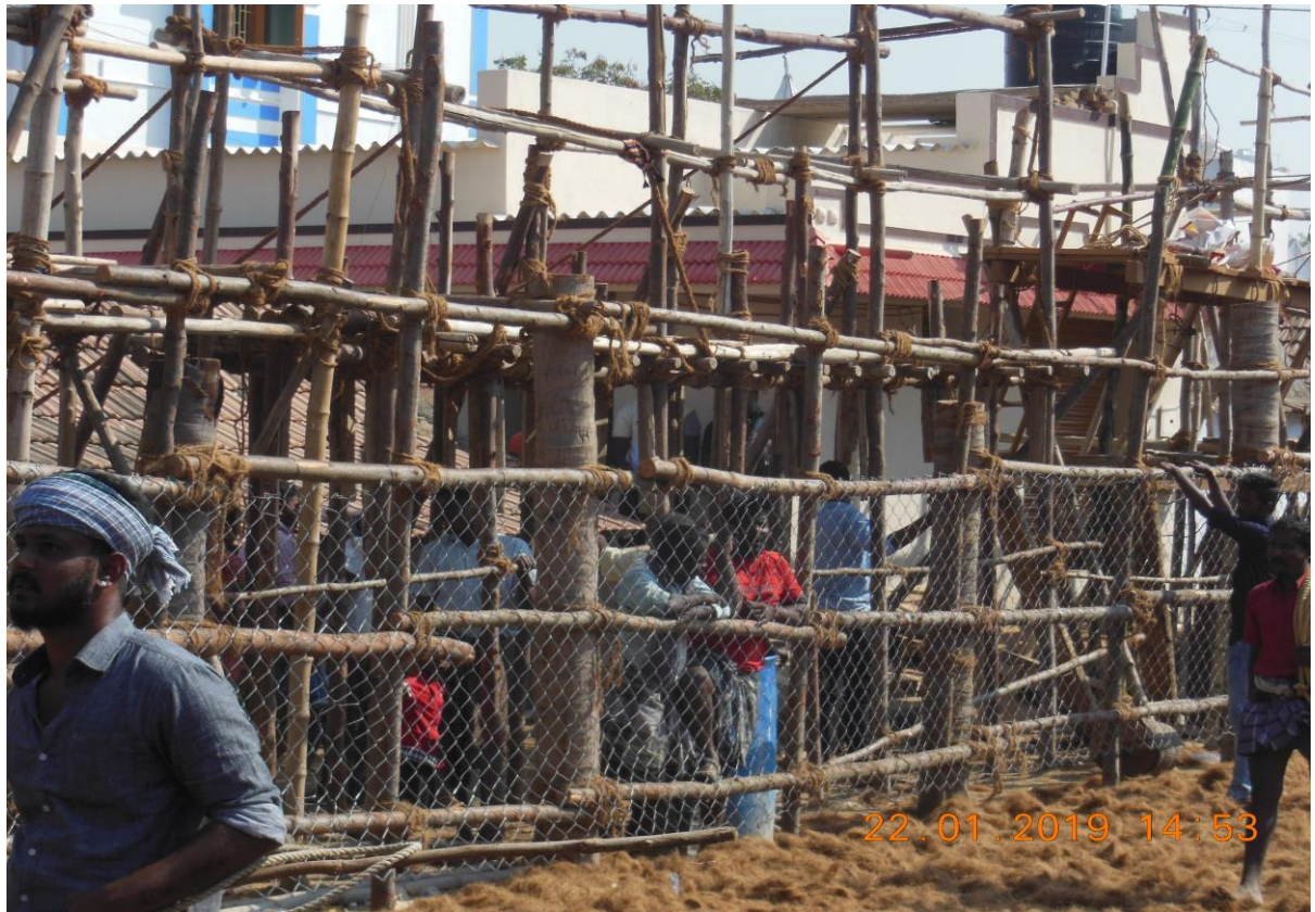
Photo 82: Barricades were less than 20 feet high in the arena, and there was no double-barricading.
